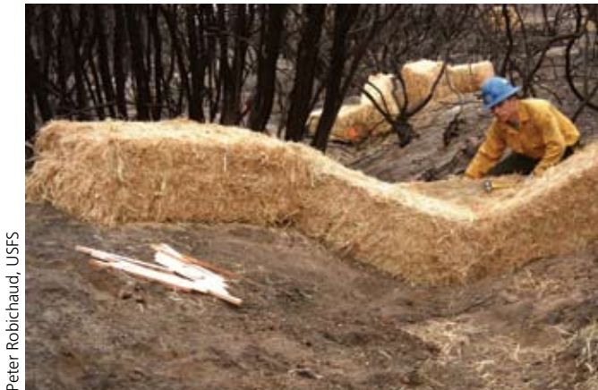
FIGURE 6.12B Straw bale check dams on a small channel within the Hayman fire.
